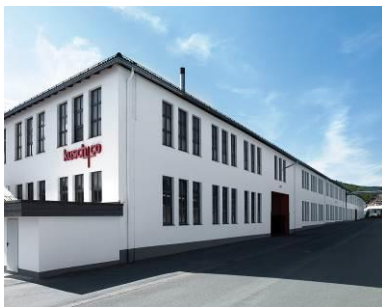
Factory 1. Administration, production of Wooden-frame seating and tables.
